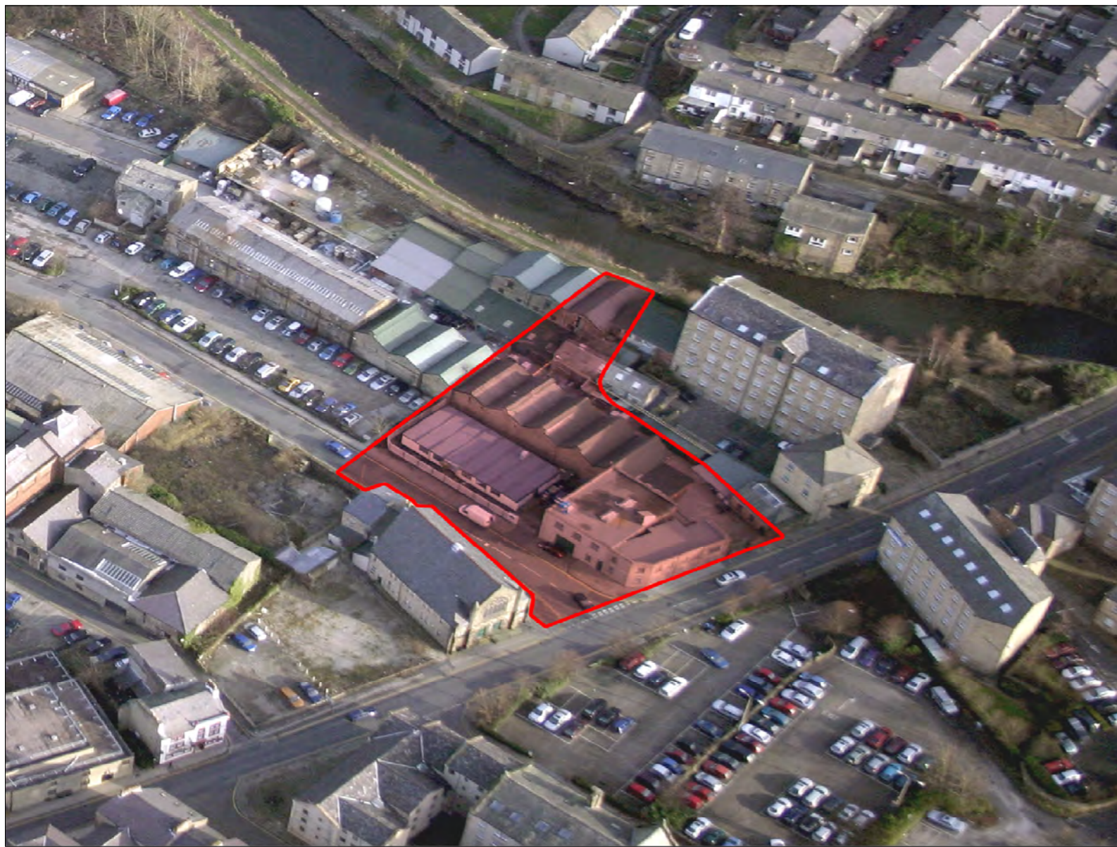
VIEW 1 - AERIAL VIEW OF EXISTING SITE
