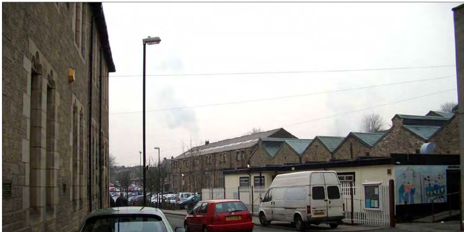
VIEW 2 - MOOR LANE TO EDWARD STREET
